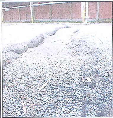
The fault line that runs through the Hohepa property.
