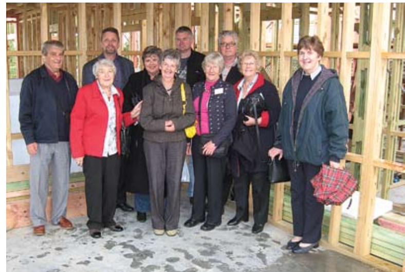
Family members of residents visit the Bev Morrissey House construction site (from left): Stan King, Raymond Eberhard (General Manager, Hohepa Canterbury), Pauline Valentine, Maree McKernan, Judy Baillie, Kevin McKernan, Gendy Brown (Hohepa Canterbury Regional Board member and Fundraising Committee Chairperson), Roger King, Shirley King and Bev Henderson.
